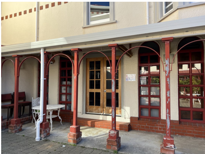
Outside of our new Parish Office
